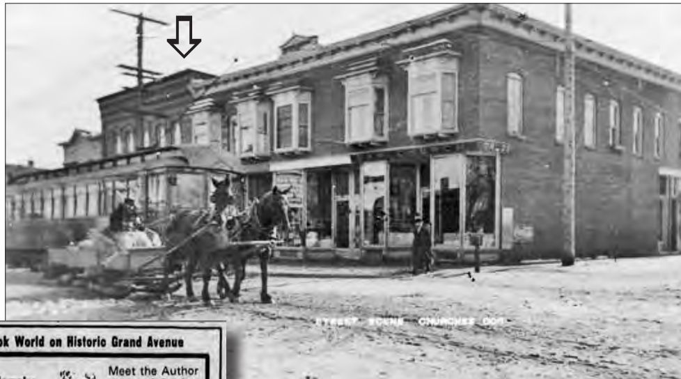
West Grand Avenue, looking east (to left)
