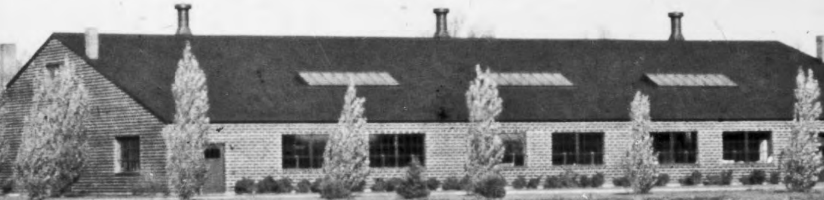
Then-new warehouse with cranberry beds in foreground
