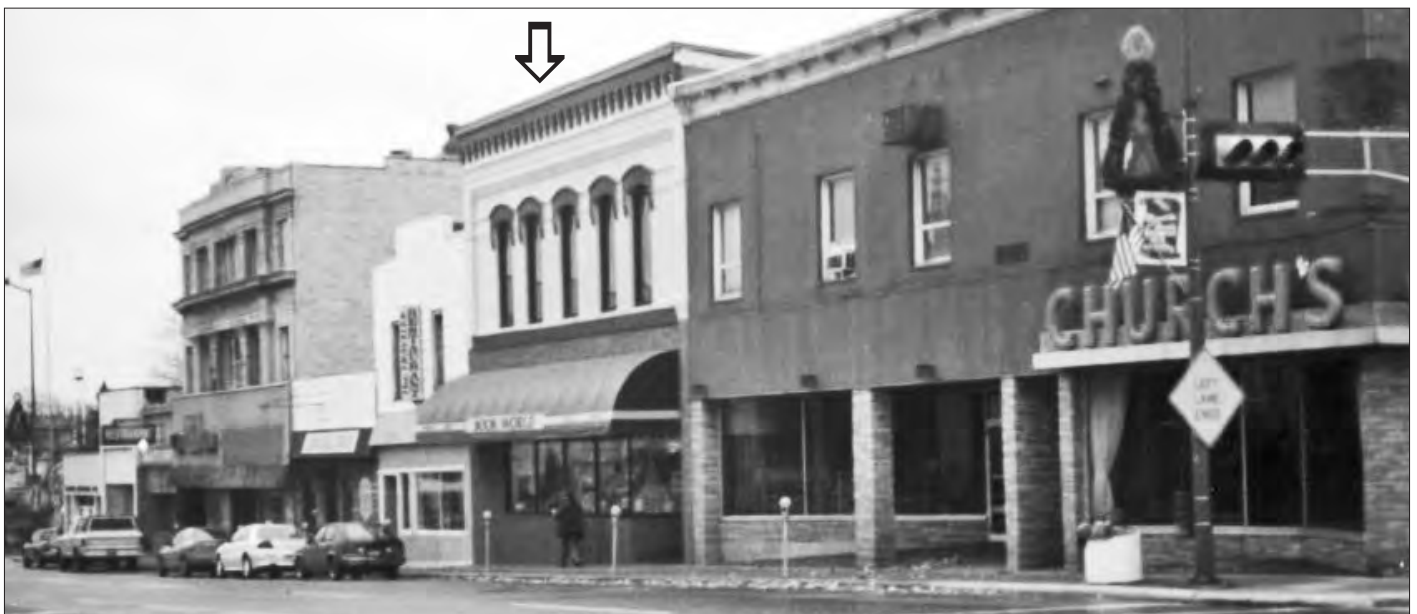
West Grand Avenue, looking east (to left)
