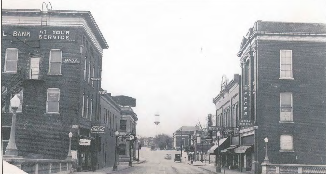
East End of Grand Ave. Bridge
