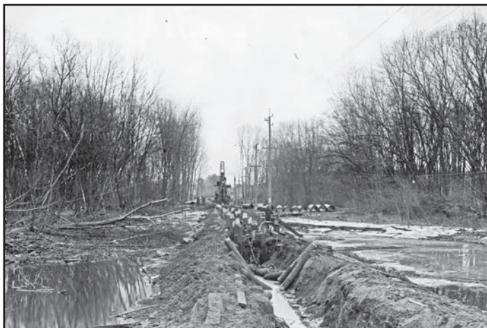
Pipeline to Port Edwards as it crossed the island swamp. Note white capped pilings and pile driver in background.
