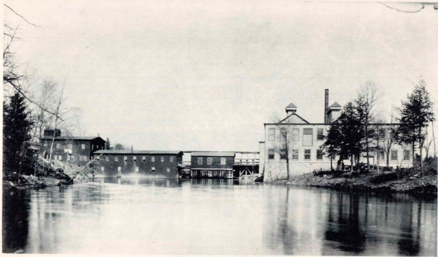
CENTRALIA PULP AND WATER POWER COMPANY.
