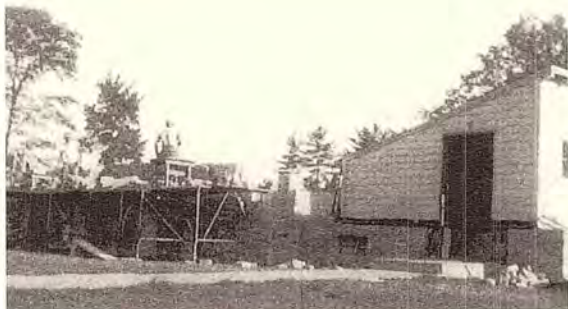
For several years, Trinity Lutheran Churchgoers used this entrance to enter the basement chapel of their church. Meanwhile, the church was being built right over their heads.
