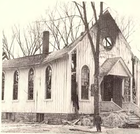
The Community Methodist Church the morning after a fire did considerable damage to the structure. The basement was salvaged and used for a few years until a new church was built.
