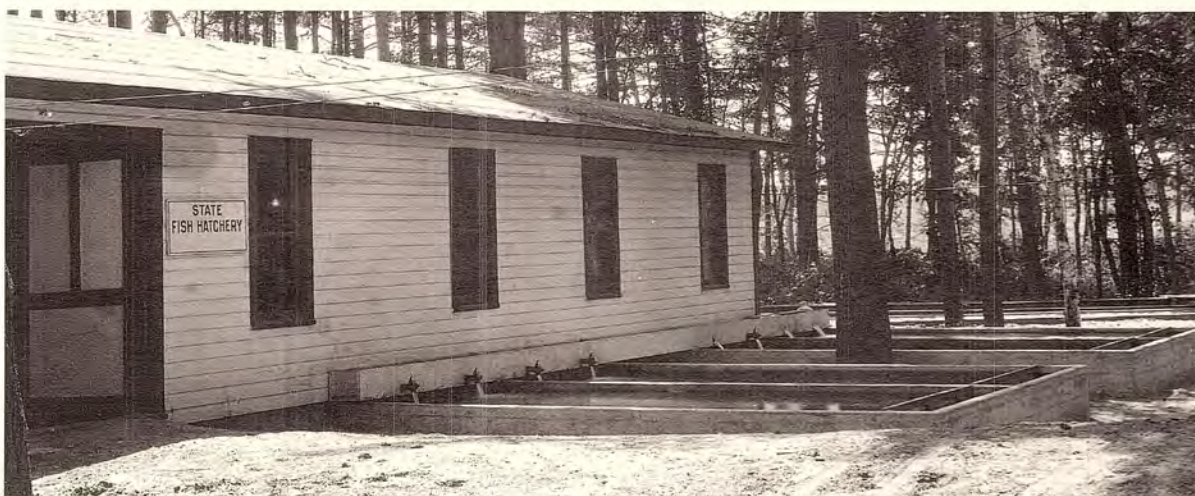
The state of Wisconsin established a fish hatchery at Nepco Lake just to stock the lake with fish. It was located near the present Nepco Lake pumping station.
