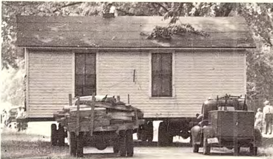
It's moving day in the village, as several homes located along Second Street are moved to new locations. House moving was more common years ago than it is today.
