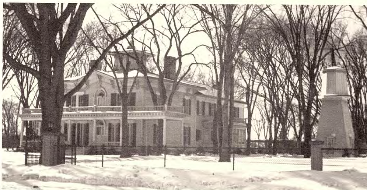
After many renovations made by L.M. Alexander, the Elm Court residence of John Edwards looked like this. It was later converted into apartments prior to demolition.
