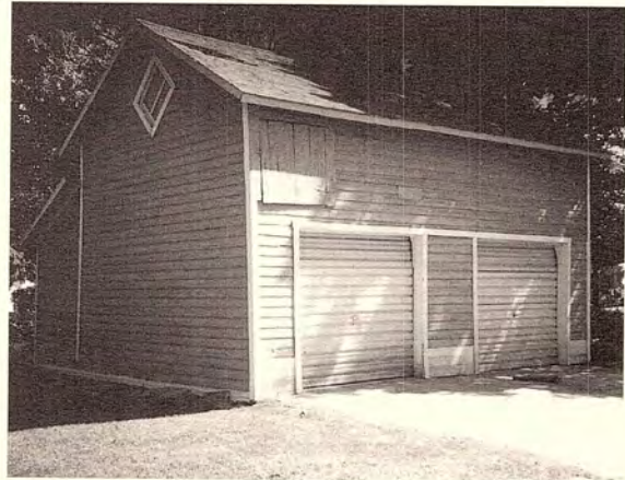
Originally a horse-and-wagon barn, there were a dozen of these structures in the village in the pre-auto era. Note the small overhead door for throwing hay into the loft. Some still stand, converted into garages such as this one.
