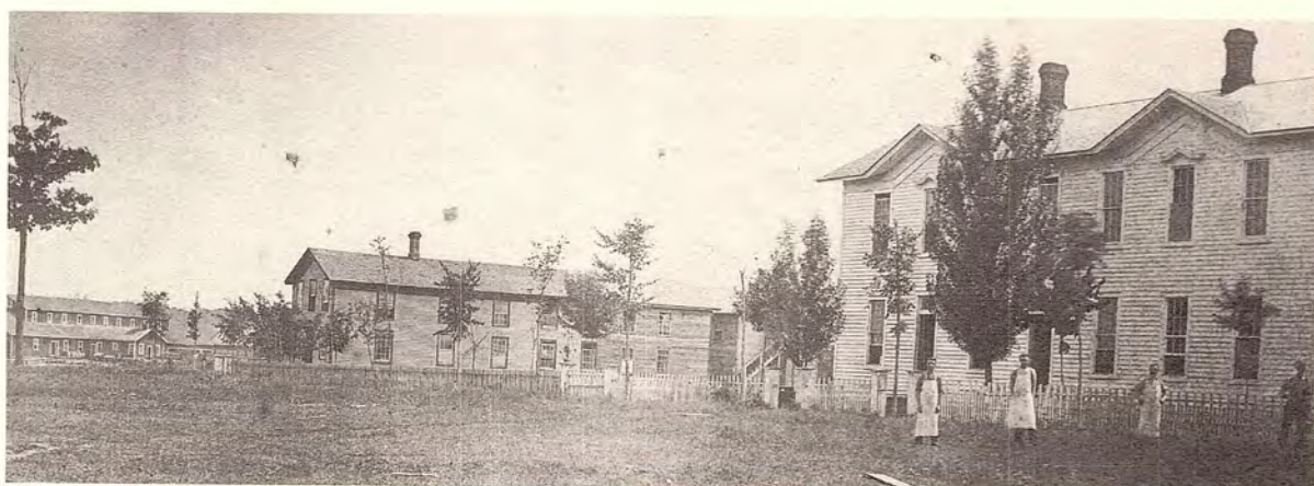
A rare old photograph showing the Port Edwards Hotel on the right. The building in the center is the annex, later moved adjacent to the hotel. On the extreme left is John Edwards' sawmill.
