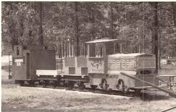
The Nepco Lake Limited, built from the construction train shown above.
