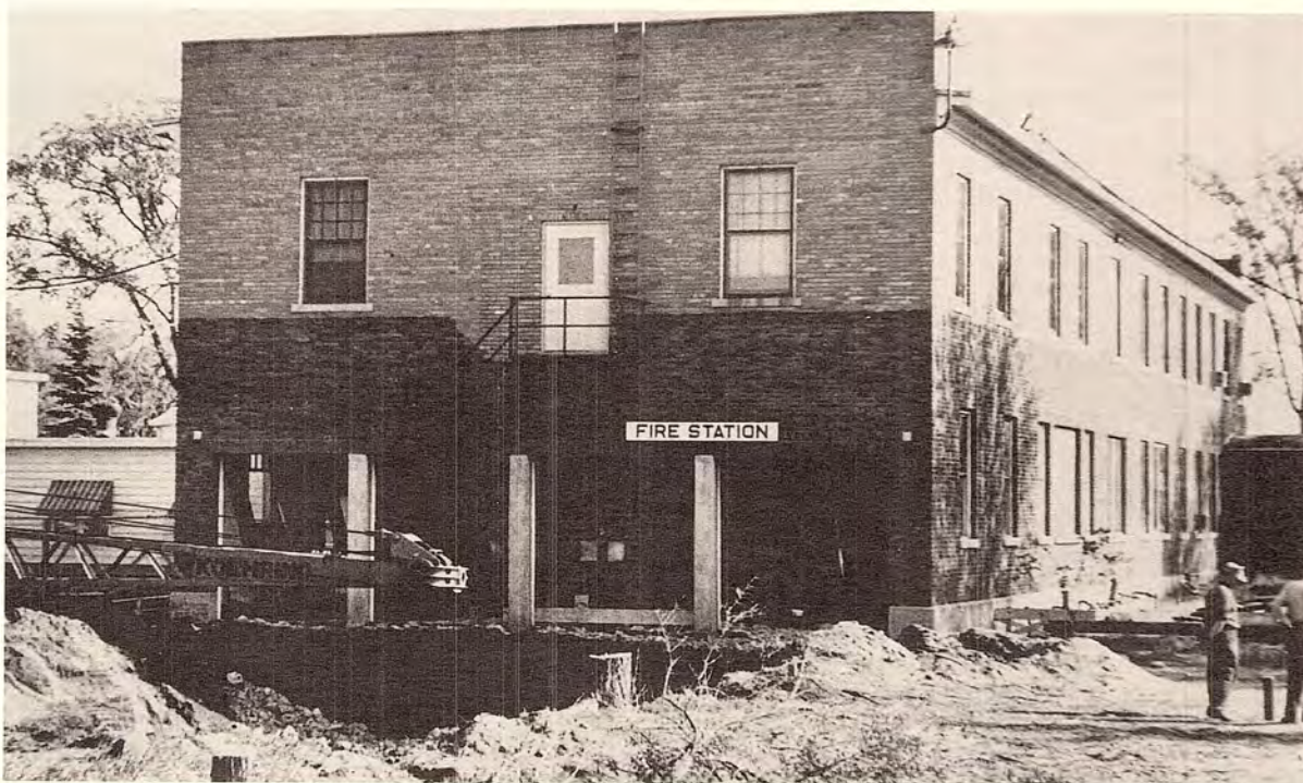
For years, the fire station was quartered in the mill office building. Here, the garages are being converted into a new NEPCO laboratory. A new fire station was built about 200 yards west of this.
