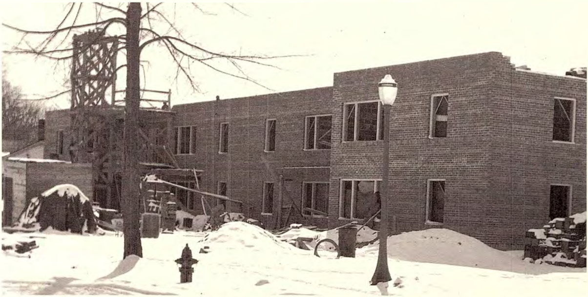
NEPCO Court Apartments are under construction as shown here. The building is being erected on the former site of the village band stand, Randrup's root beer stand, and the village hall.
