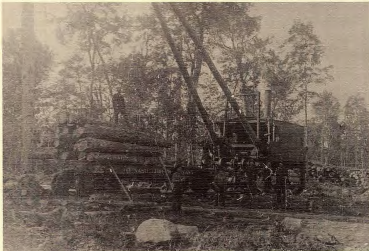
A McGiffert log loader working on the Nash property in Northern Wisconsin, somewhere along the rail line of the Glidden and Southwestern Railroad. The logs were destined for the sawmill at Shanagolden. The railcar carries the name of the Nash Lumber
