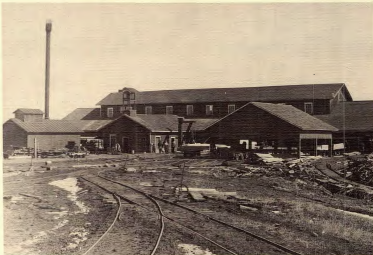
The lumber mill of John Edwards and Company was located on the same site occupied by the present Port Edwards mill. The railroad tracks in the foreground were not common carrier tracks but only an intramill system used for transporting lumber from
