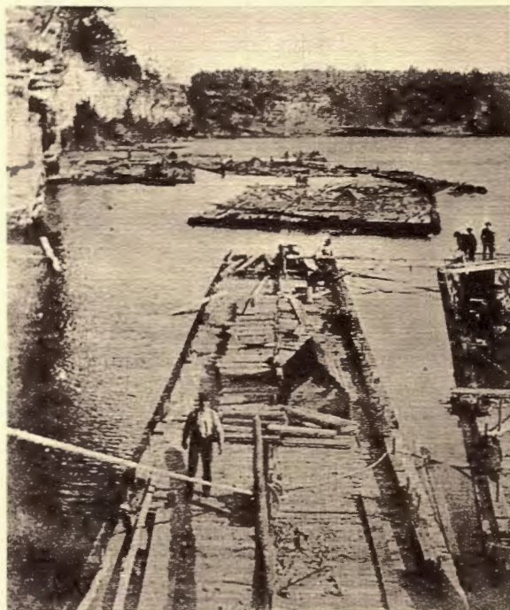
Lumber rafts congregate at Kilbourn Town (Wisconsin Dells), prior to going through the narrows of the Dells. The raft in the foreground is being separated into what is called a rapids piece. In the background are rafts that have come down the river from Port Edwards, Grand Rapids and other points further north on the Wisconsin River.
