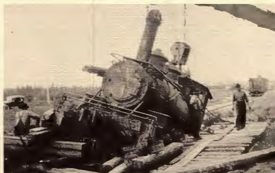
Not only is the only locomotive of the Glidden and Southwestern Railroad out of service but the main line is also fouled up. The derailment was caused by a soft roadbed in the marsh area between Shanagolden and Glidden, Wisconsin.
